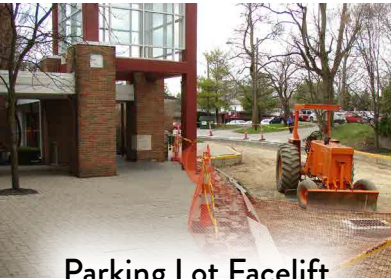
Parking Lot Facelift
